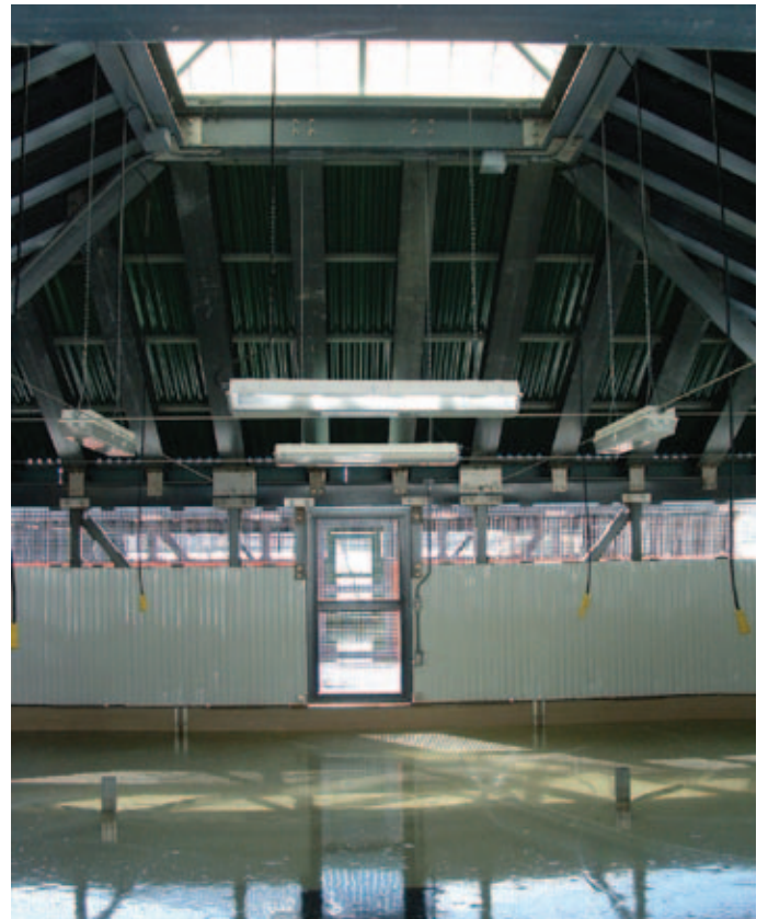
The Craig Brook National Fish Hatchery in East Orland Maine used corrosive-resistant EXTREN® structural shapes to frame roofing structures over moisture rich crowding pools.
