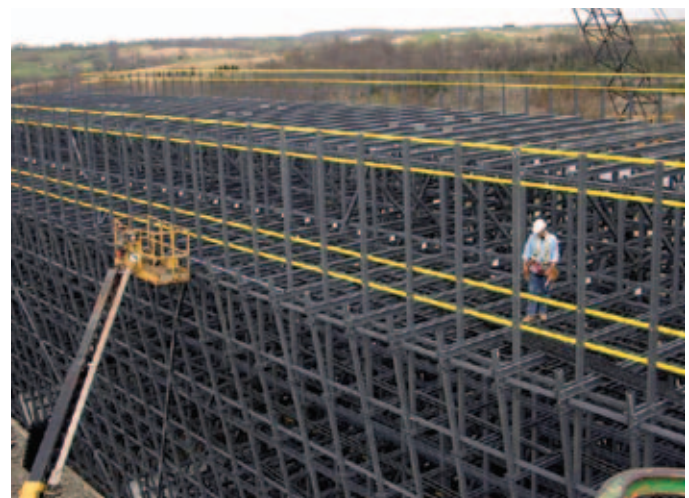
EXTREN® does not rot or corrode, making it the ideal material for cooling tower construction.
