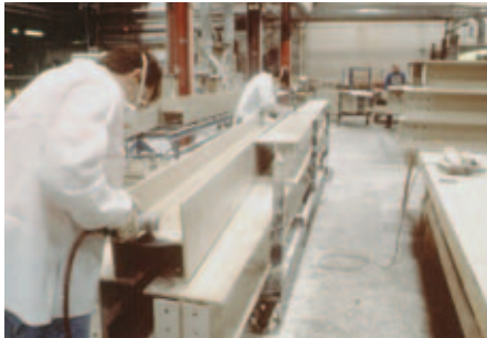
Beams are prepped before bonding connections together.
