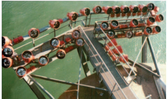
EXTREN® structural shapes were used to fabricate twelve platforms holding the spotlights that illuminate the Forth Bridge in Scotland.
