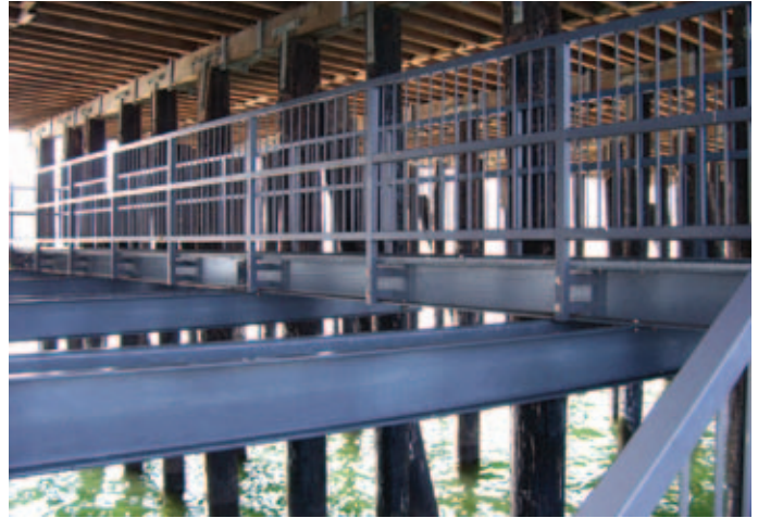
The Avila Beach Pier in California was reconstructed using EXTREN® structural shapes for support, DURADEK® pultruded grating, stair treads and handrail.
